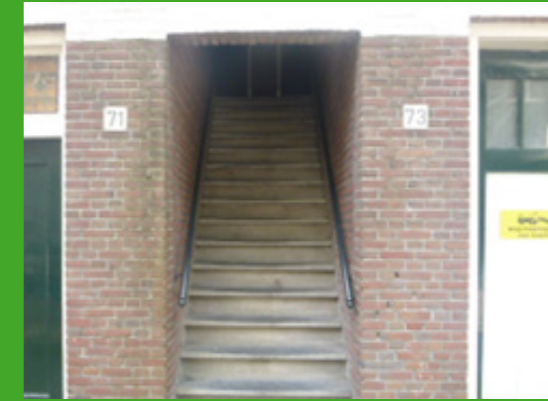
Foto 32: coating op trapleuningen (lood)
