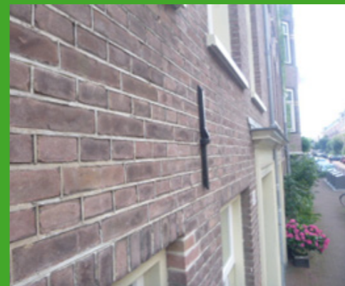
Foto 33: coating op muuranker (lood)
